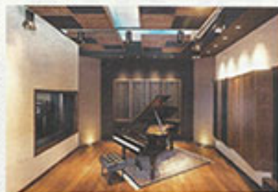
Valenzo's live room is spacious, and acoustically malleable via movable panels, with an adjustable RT60 between 0.7 and 1.2 seconds at 1 kHz.
